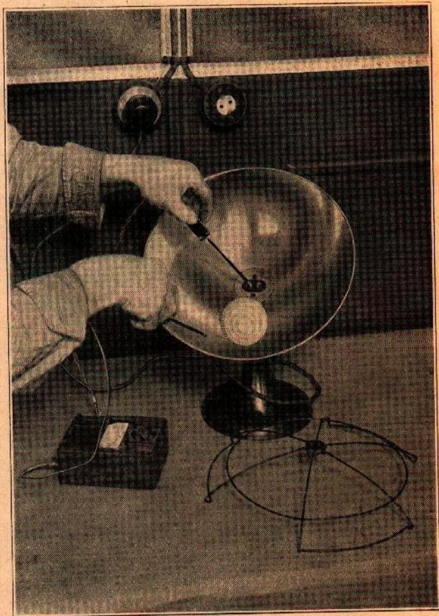
Figure 15. Measurement of continuity from the frame of a bowl fire to earth, as described on Page 27. Element removed for convenient access to terminal.
