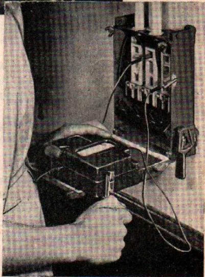
Figure 11 wee-Megger test on an installation
